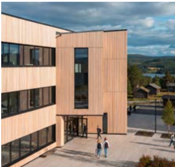
In schools, reducing impact sound between floors and classrooms helps maintain calm, focused learning environments.
