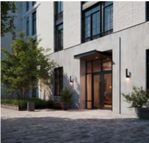
Multi-occupancy buildings are required to meet defined standards for noise control to ensure appropriate acoustic performance.
